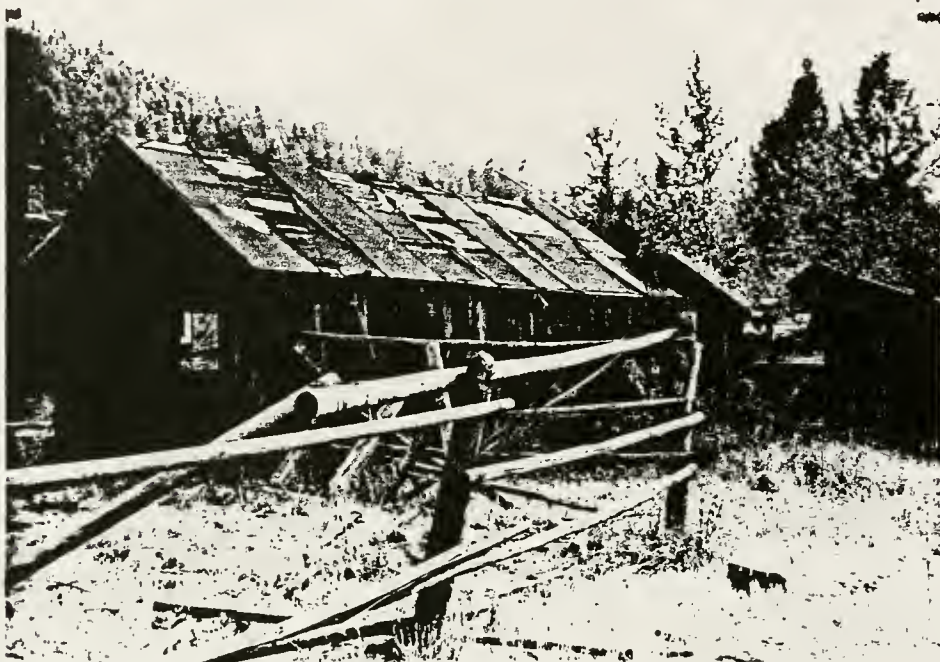
Figure 213. Structure #94, southeast view.
